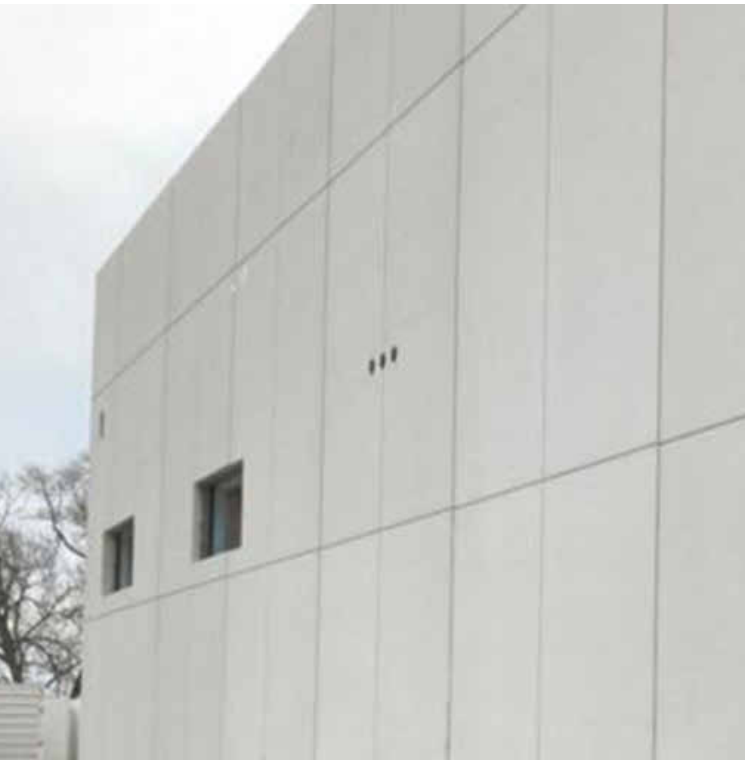
CODE: CP1 MATERIAL: PRECAST CONCRETE WALL PANELS COLOUR: PLAIN FINISH: PLAIN FINISH
