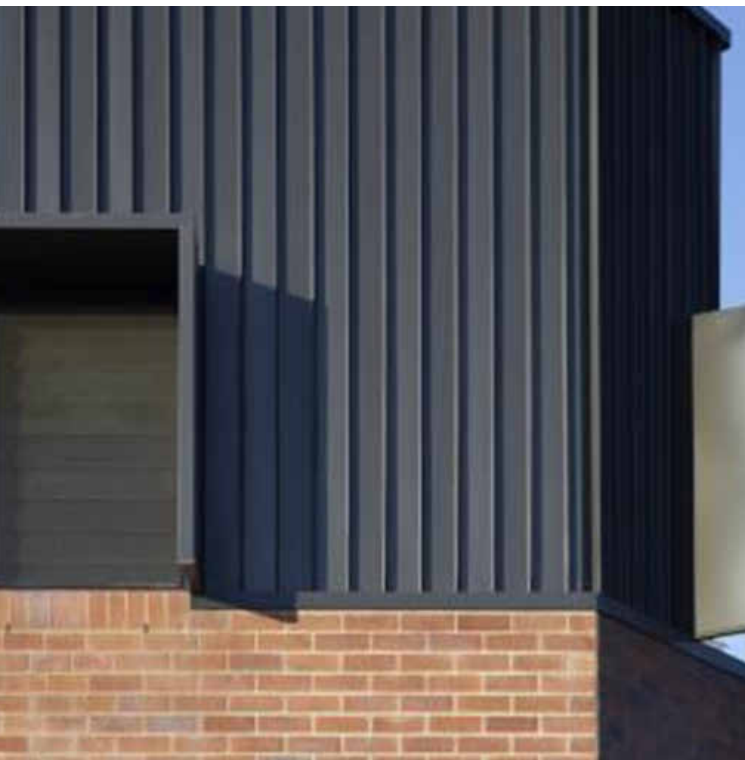
CODE: PM1 MATERIAL: PROFILED METAL WALL CLADDING COLOUR: DARK FINISH: PROFILED
