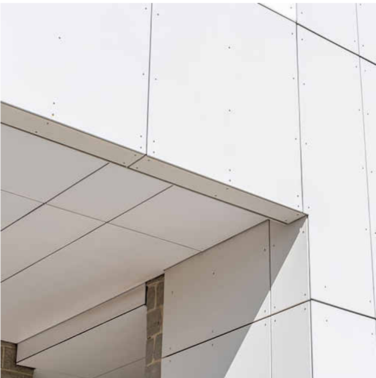
CODE: FC2 MATERIAL: FIBRE CEMENT CLADDING OR SIMILAR COLOUR: WHITE FINISH: PLAIN PANELS WITH EXPRESSED JOINT
